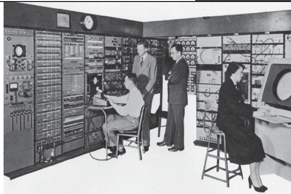
Whirlwind: early graphics using Vector Scope (1951)
